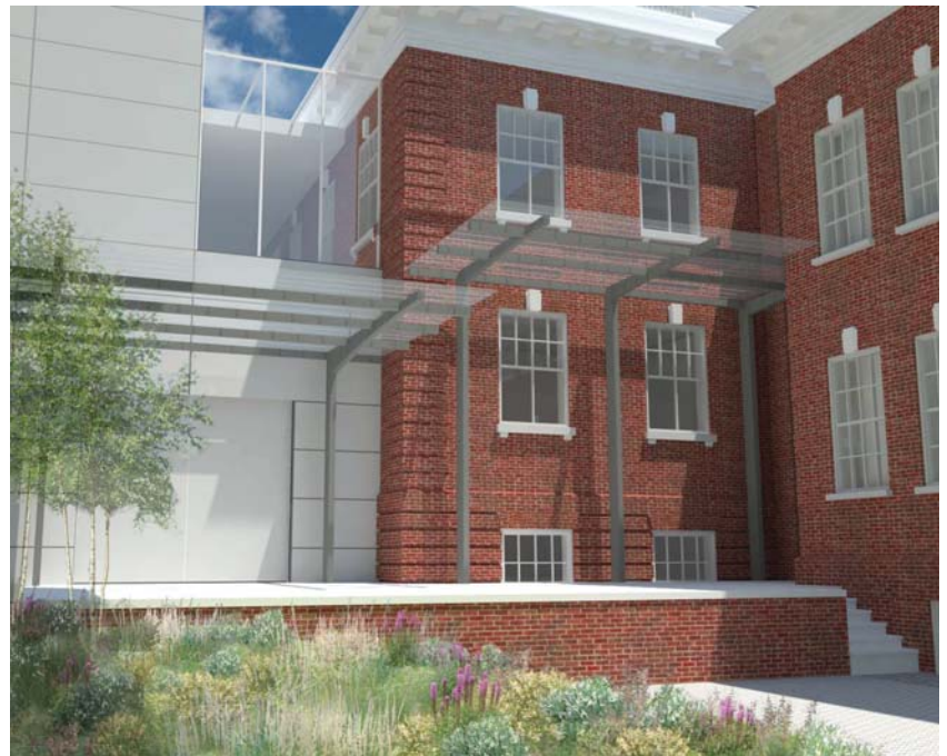
LOADING DOCK AT MUSEUM
